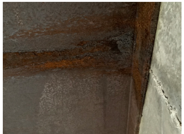
1st joint , upstream right, on inside
