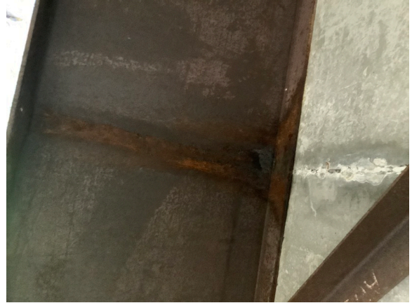
1st joint, upstream right side
